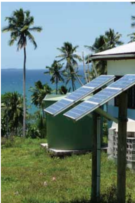
Health centre with solar power in Sanma Province, Vanuatu.
